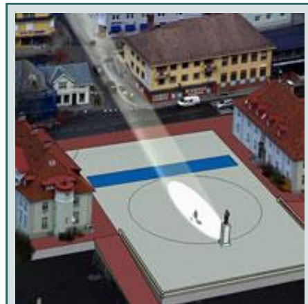
Sun-tracking mirrors capture sun rays and direct them down to the center of Rjukan, Norway (Image Source: visitnorway.com)
